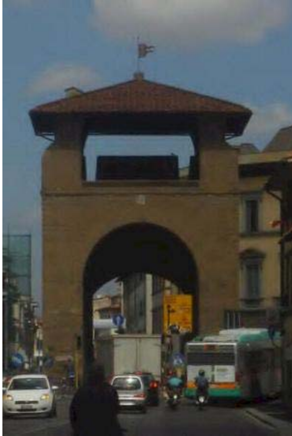
Guadagni Palace of Porta a Prato, two windows, 1 st and 2 nd floor, are visible on the right, behind the Medieval City Door of Porta a Prato.
